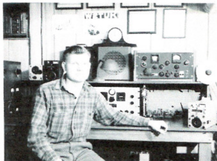
Harry Dannals as W2TUK in 1947 at age 19 in the station he shared with his dad, W2GG, using an ARC-5 converted military transmitter for 80 meters and a BC-779 (WWII version of the Hammerlund Super Pro). (Courtesy: Harry Dannals W2HD)
