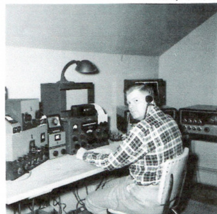
W2TUK in the attic shack at his first home with his wife Kay in Bethpage, on New York's Long Island. On the bench: a Johnson Viking II transmitter with VFO, a Collins 75A4 receiver, and Johnson MatchBox that fed a 40 meter dipole. (Courtesy: Harry Dannals W2HD)
